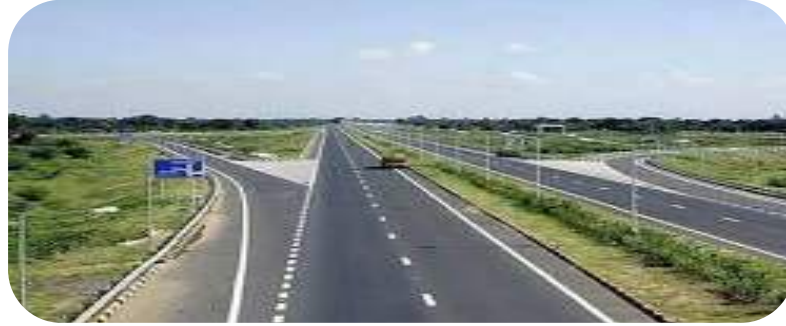
The Nagpur-Mumbai Super Expressway
